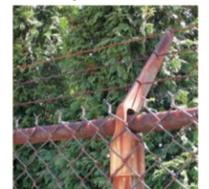
Corrosion can be dealt with by cleaning the affected joint, insulating the junction so electrical contact is no longer made, or by making a solid electrical connection between the offending parts. Some fences or galvanized structures may need to be removed or replaced.
